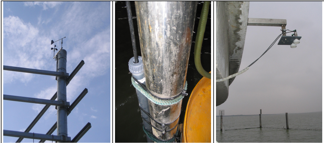
Figure 4 Instruments installed at Gonghu: anemometer and wind vane (left); pressure gauge (centre) and Log_aLevel (right; source photos: RWS, 2006)
