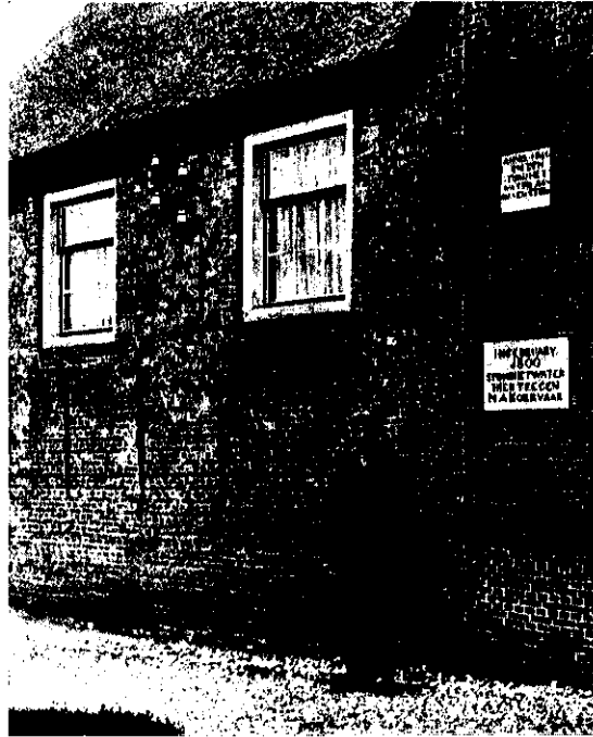
So-called water stones in old Dutch farms tell the tale of disasters. The farm here has five rooms, each floor about 4 feet higher than the preceding one. When the floods came the family moved to the necessary height. The cows were put in their roof stable about 15 feet above the fields. The farms were protected against waves, floating beams and ice by means of floating willow mattresses, which the farmer 'wove' around the building before the flood came.
