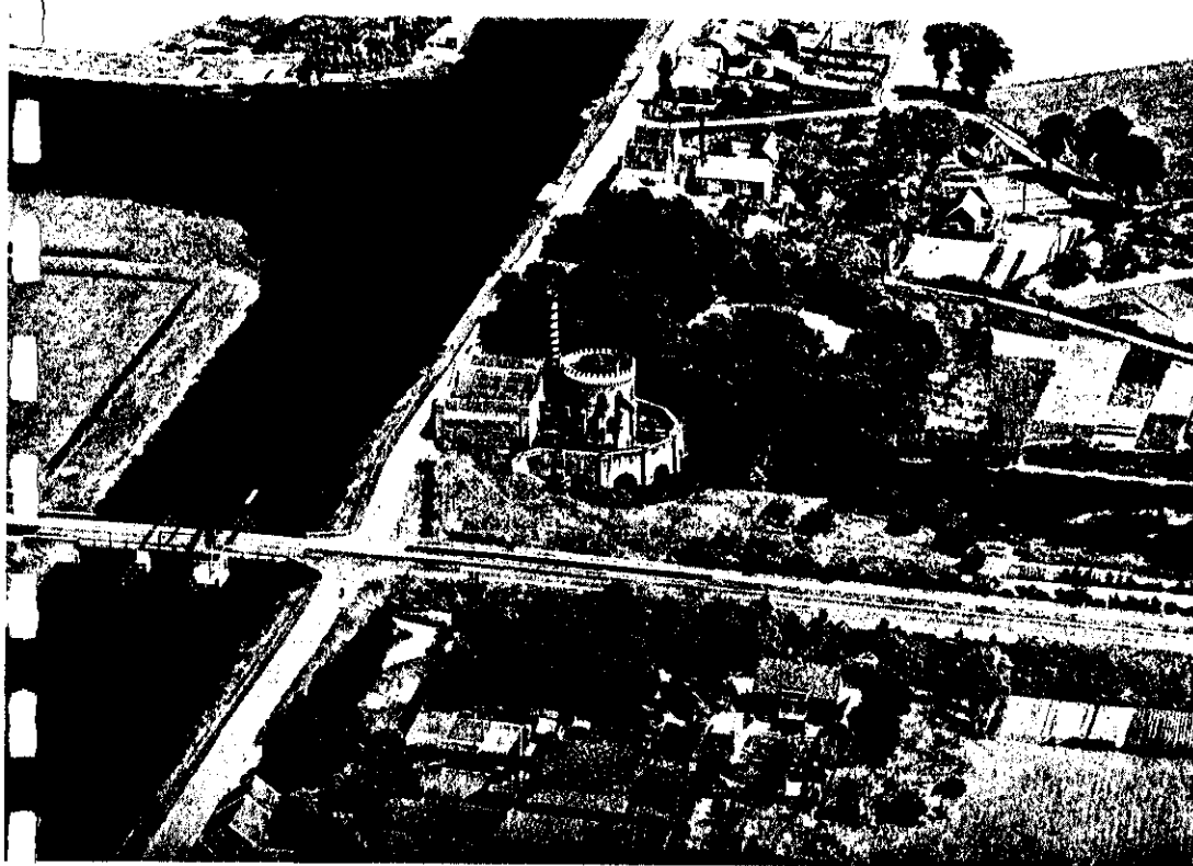
(Photo K.L.M.) The Cruquius pumping station near Haarlem was one of the three which pumped the Haarlemmermeer dry after some years of pumping (1852). Its machines are British, it is a museum today. The bottom of the lake can be seen in the right part of the picture. The water was pumped into the ring canal (left). Today modern pumps do the work of keeping the lake bottom dry. Schiphol aerodrome lies on that bottom.
