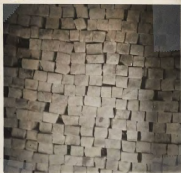
11. Steenglooijing losse zetting.
