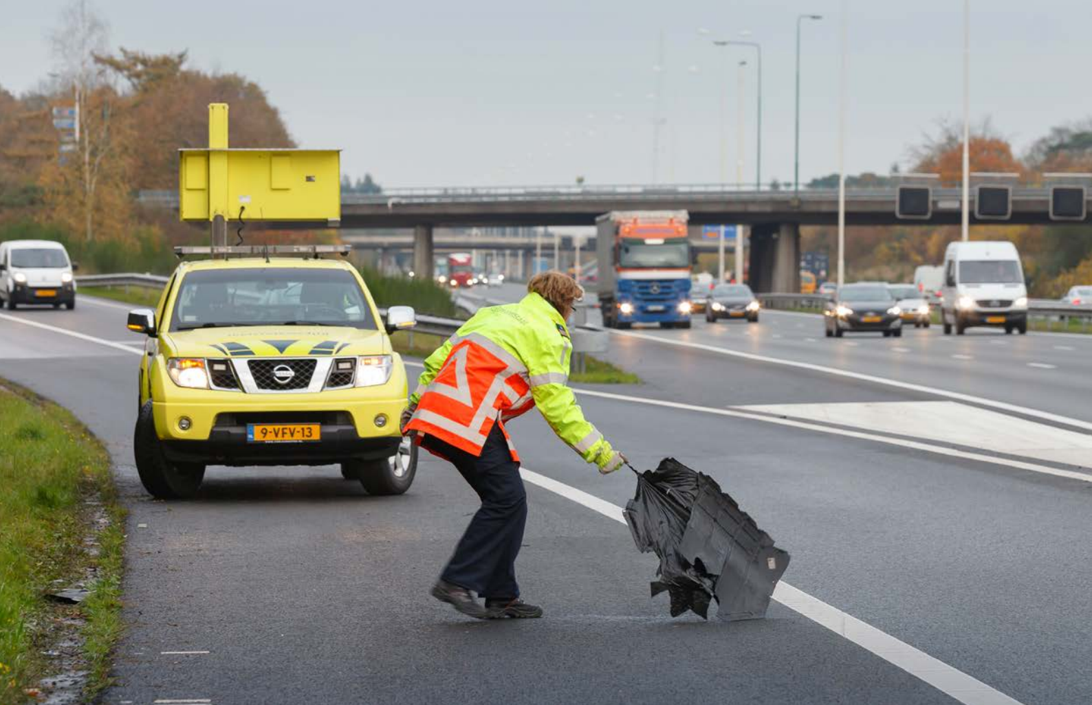
A road inspector clears the carriageway
