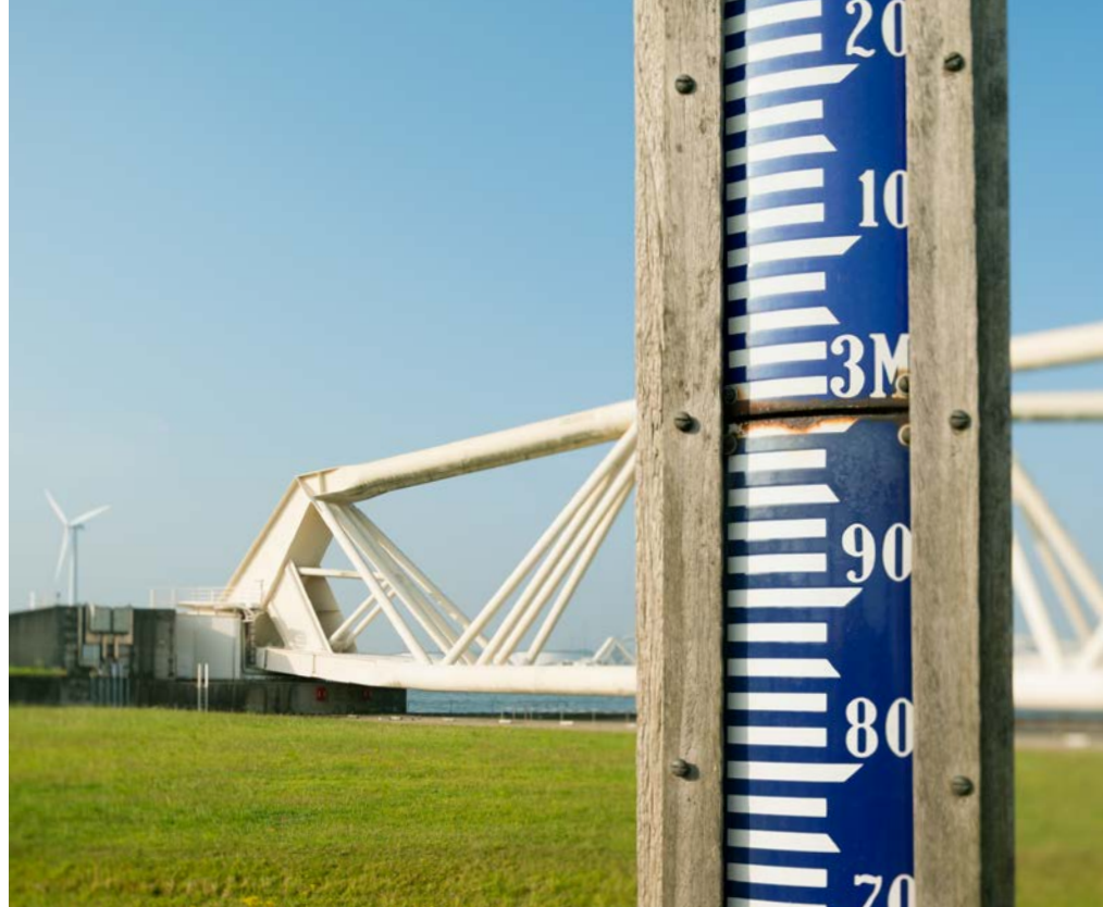
Water level meter at the Maeslant storm surge barrier
