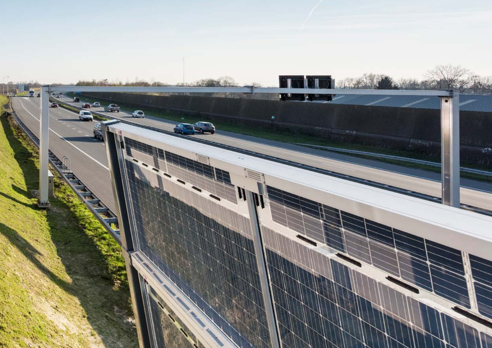
The solar highway near Uden (A50)
