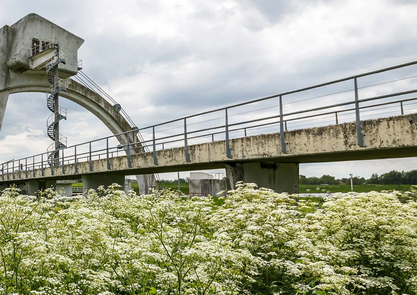
Hagestein Dam in the River Lek
