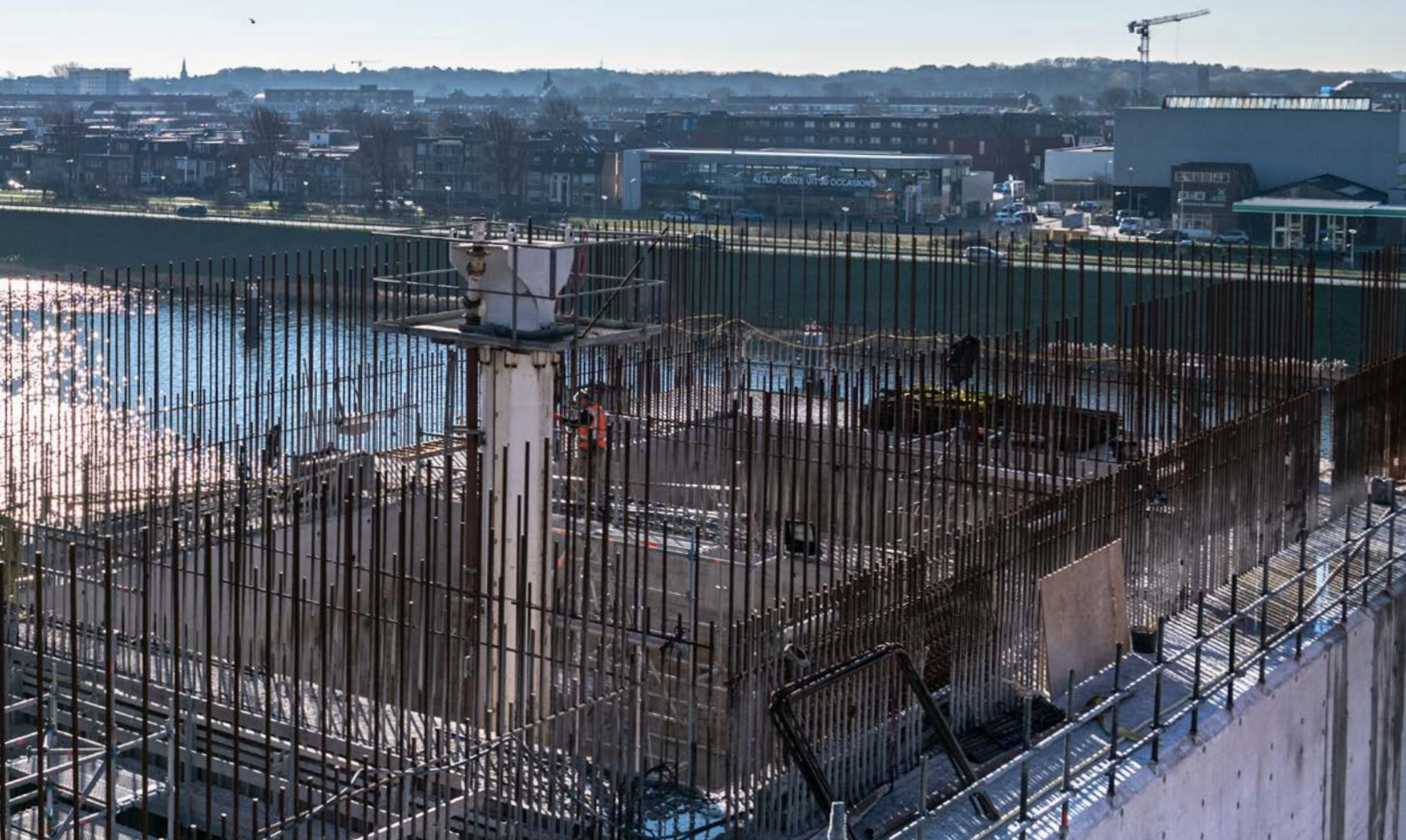
Work on the landward wall of IJmuiden Sea Lock
