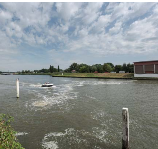
Bubble screen in the Amsterdam-Rhine Canal
