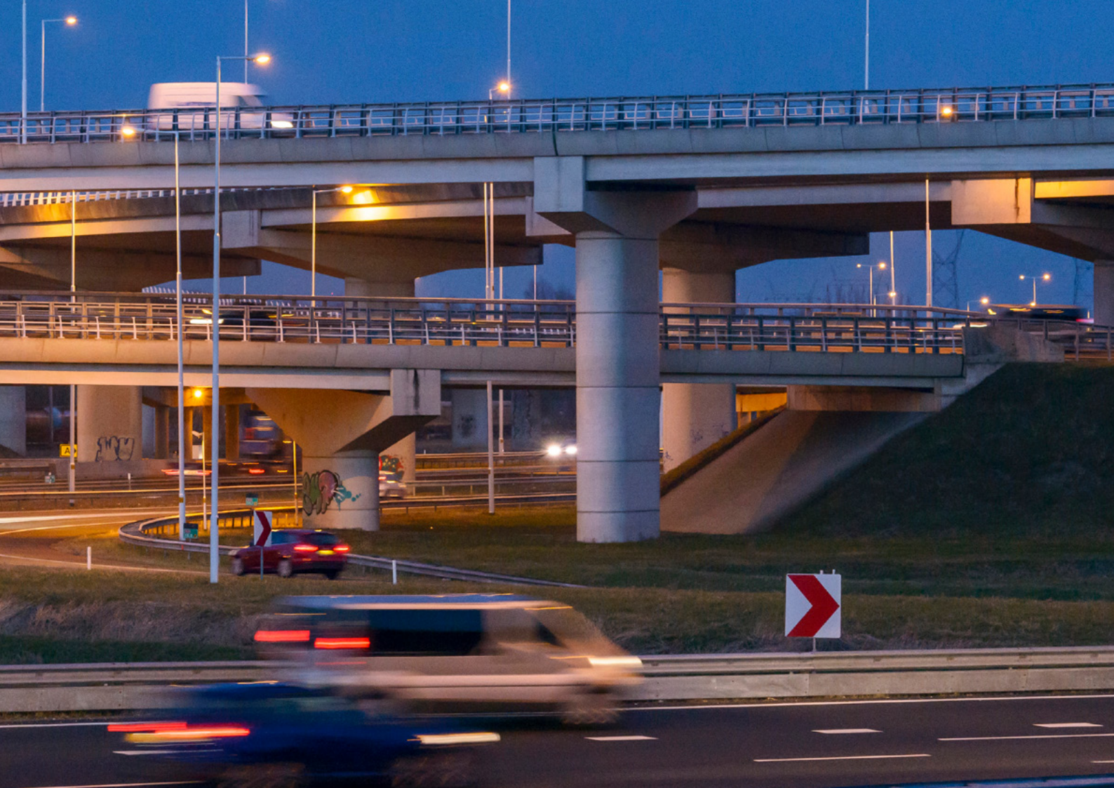
The Vaanplein intersection near Rotterdam
