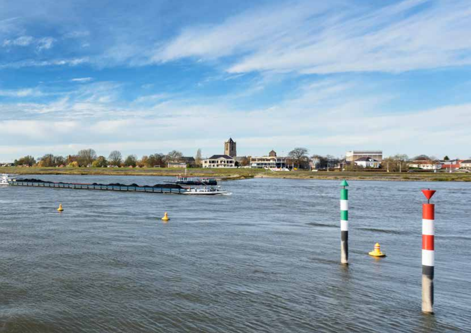
Parallel dam in the River Waal
