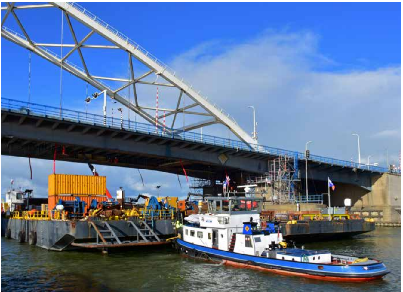
Repair work on the Merwede bridge
