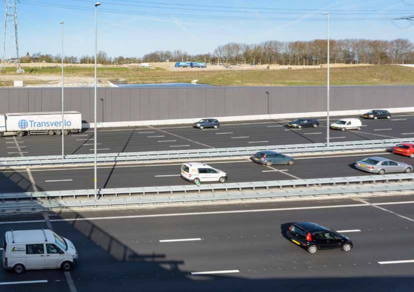
The new aqueduct and rerouted A1 motorway at Muiden
