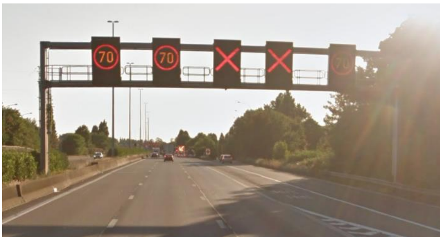
Figure 5: Dynamic lane signalling gantry, information also provided by the IVS service
