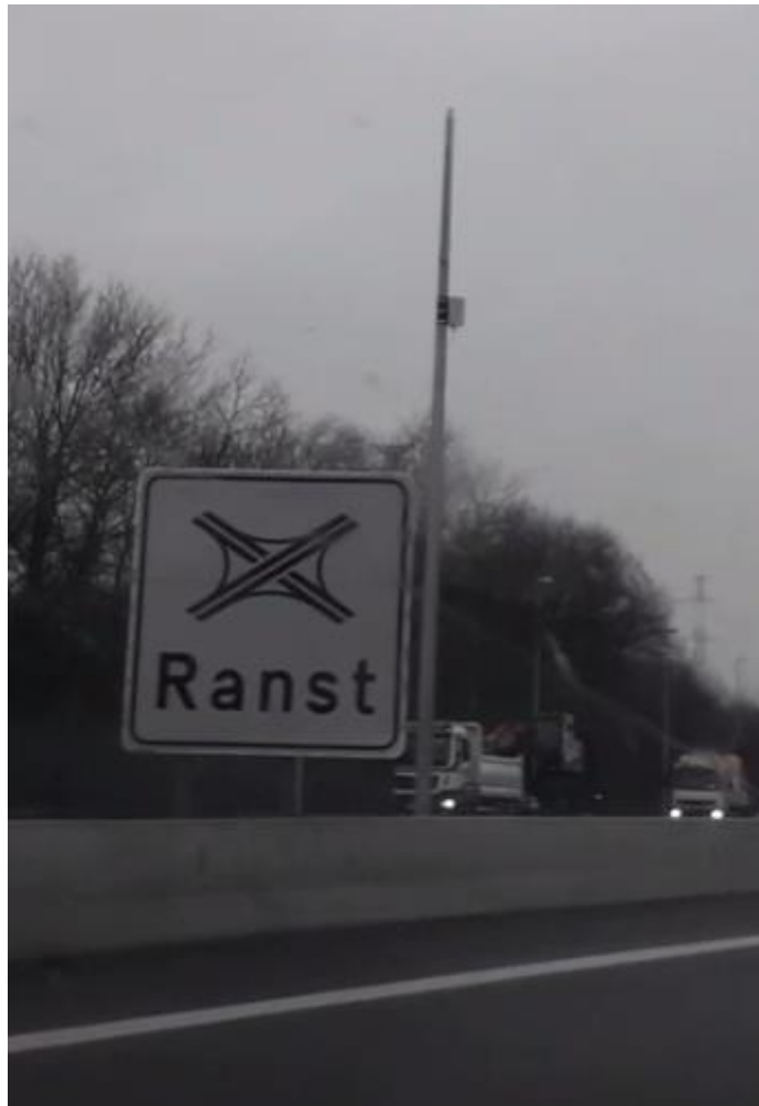
Figure 15: RSU on a pole on the E34
