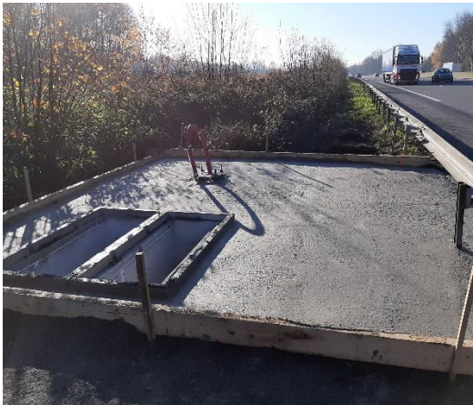
Concrete foundation for a road side unit on A25
