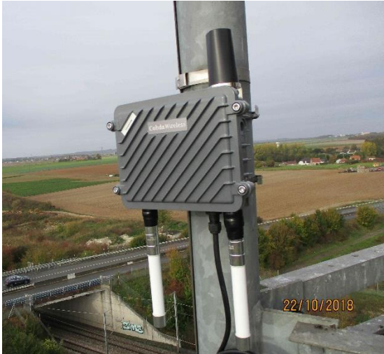
Road side unit on a pylon in Esquerchin (A1)
