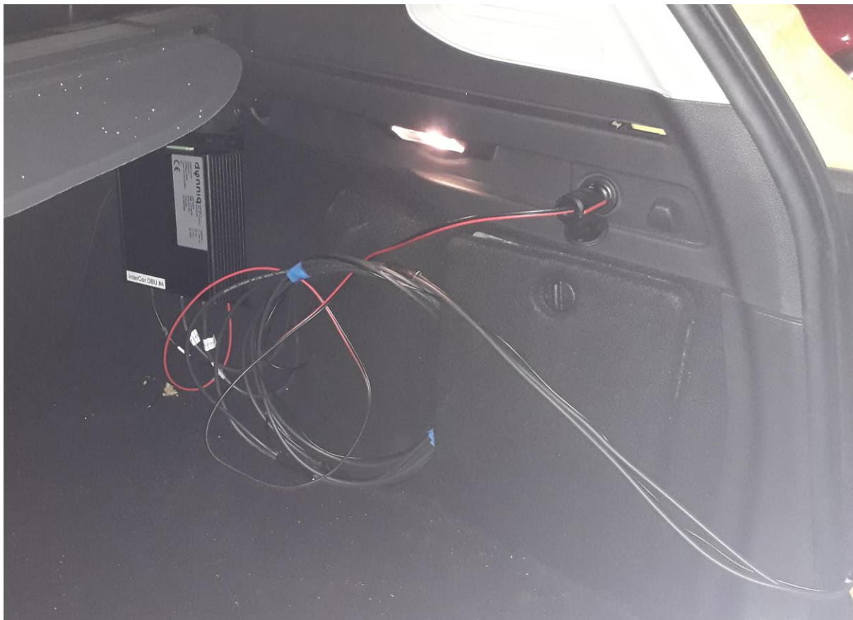
Figure 17: On-Board-Unit installed in the boot of the car.
