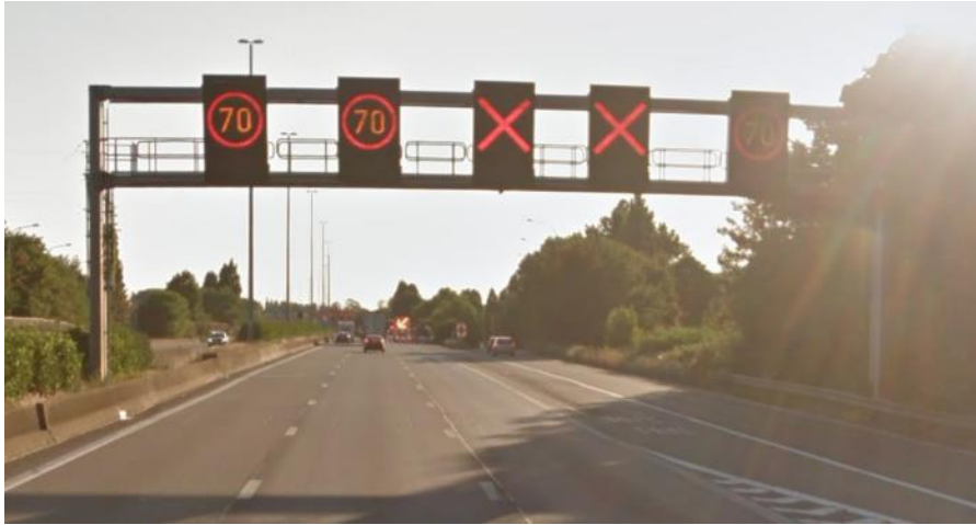
Figure 7: Dynamic lane signalling gantry, information also provided by the IVS service
