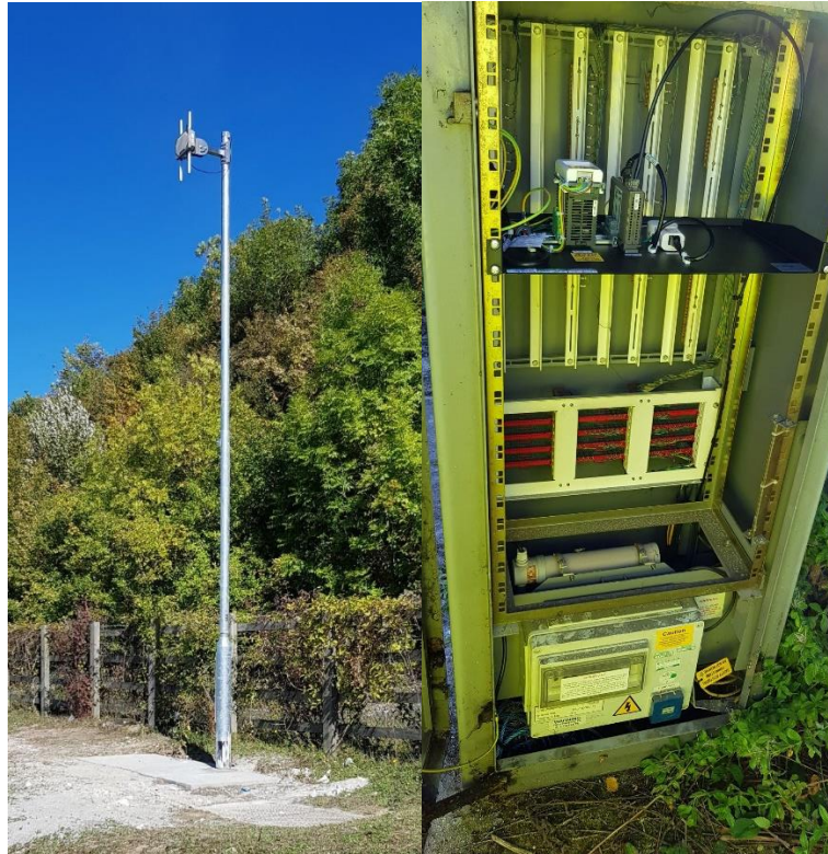
Figure 61: Short Range Deployment on A2 M2 of 32 ITS-G5 Roadside Units
