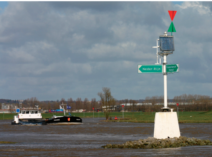
Bifurcation point ('T-junction') at IJsselkop, seen from the south. The ship is approaching from the IJssel.
