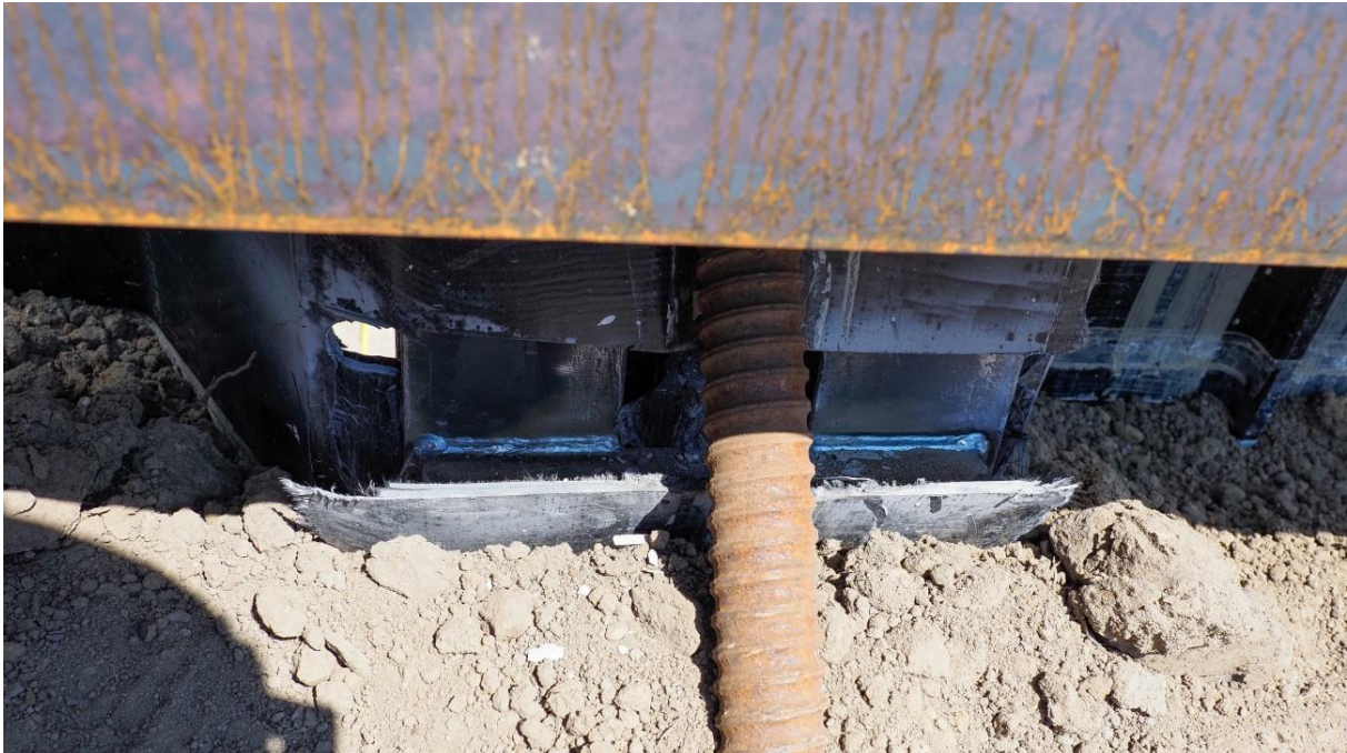
Figure 9-6 Local buckling and delamination of the outer 0/90 laminate layer
