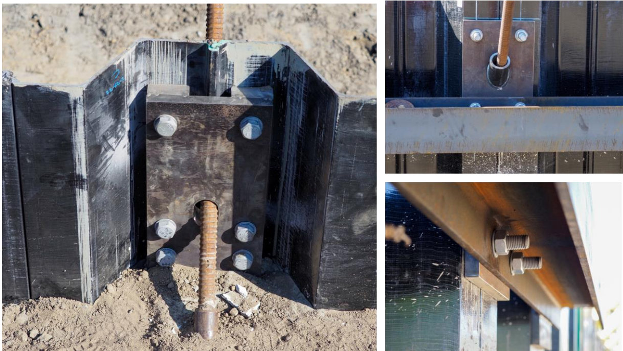
Figure 6-11 Sheet pile connection test 3
