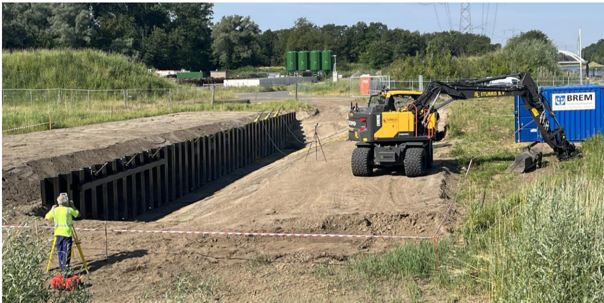
Figure 6-1 Total station+ 3 hydraulic jacks in the back
