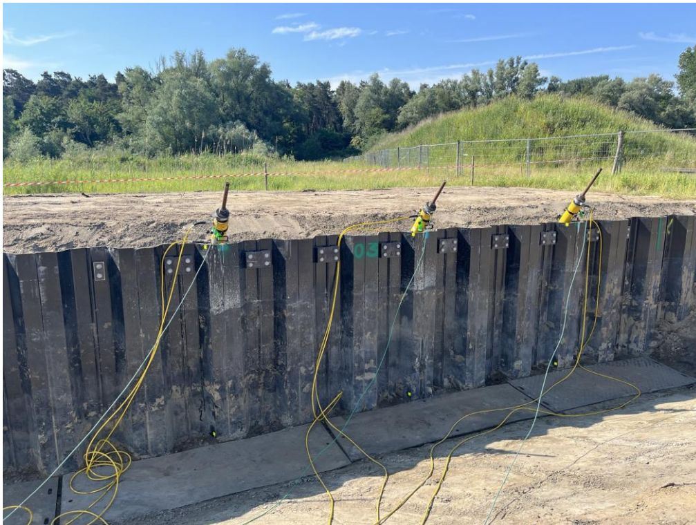
Figure 6-4 3 Set-up with the hydraulic jacks
