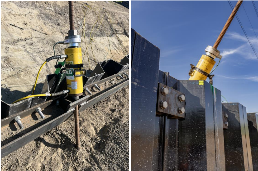
Figure 6-6 Sheet pile connection test 1
