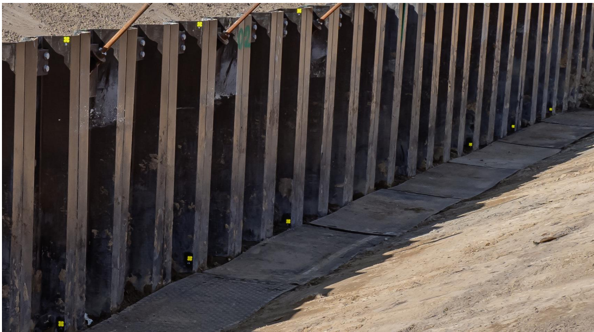
Figure 6-3 Yellow dots indicate high and low measurement points
