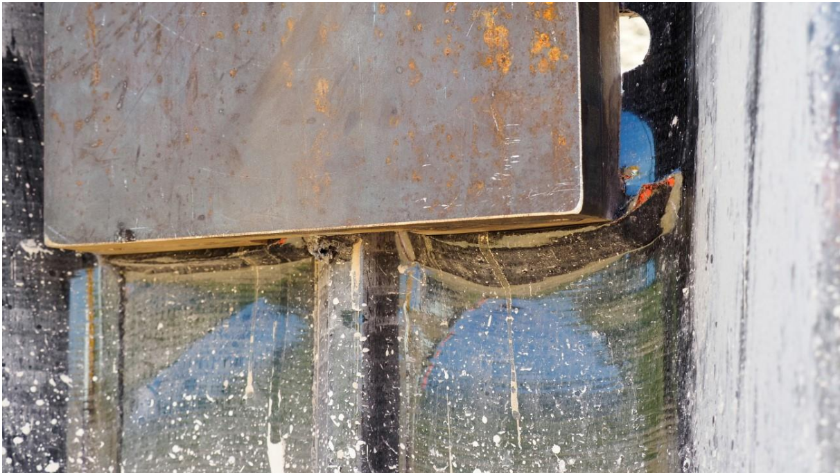
Figure 9-9 Local buckling and delamination of the outer 0/90 laminate layer
