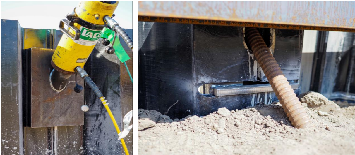
Figure 6-9 Sheet pile connection test 2
