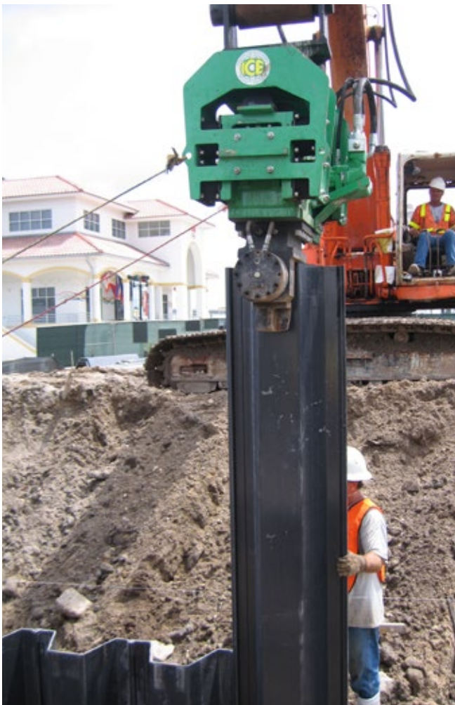
Vibratory Hammer Installation Example
