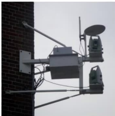
Figuur 5.6 / Robotic total station, RTS.
