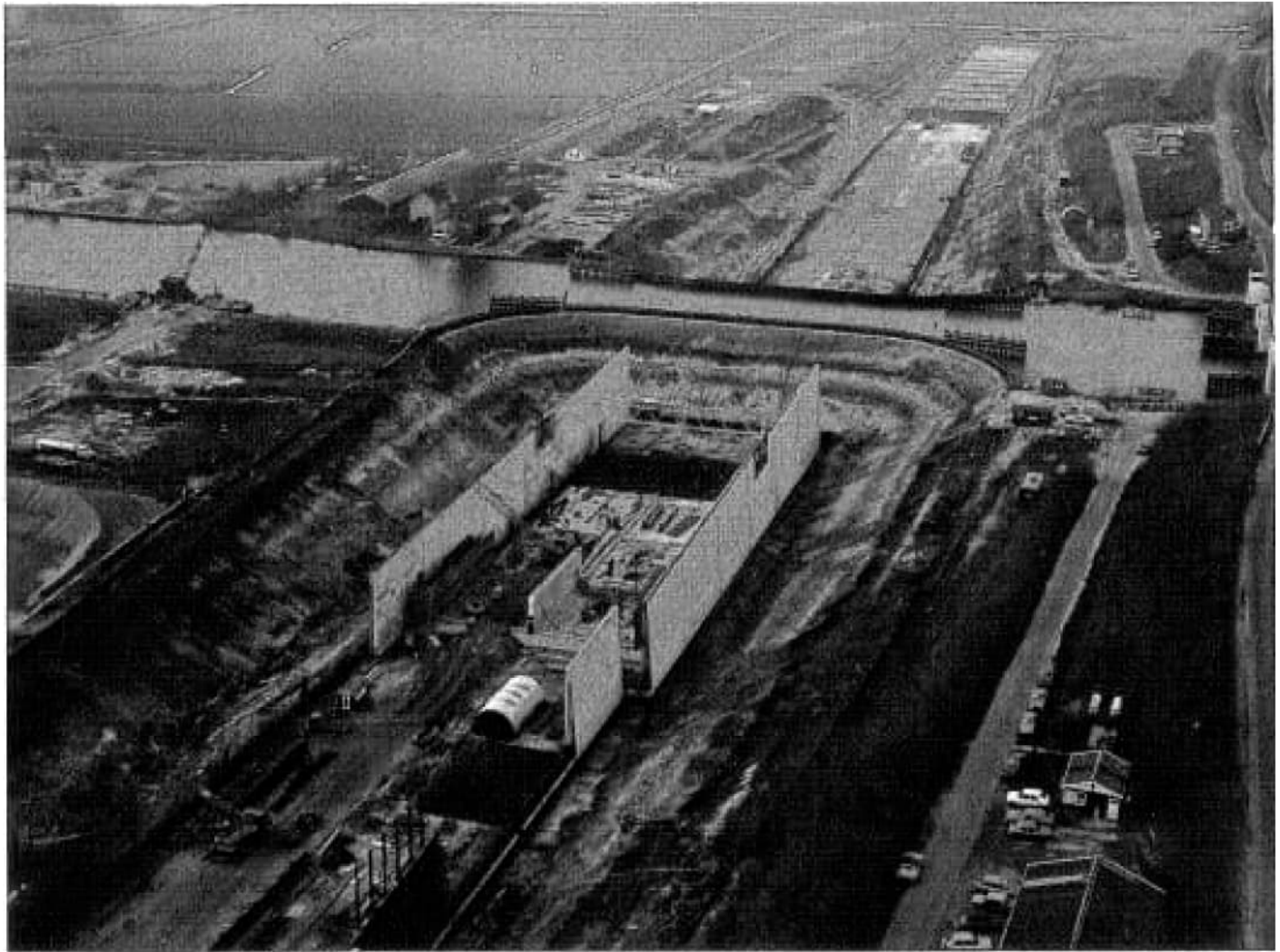
Overzicht van beide bouwputten; zinkelement is reeds in aanbouw Survey of both the building pits; tunnel element under construction foto: KLM Aerocarto BV
