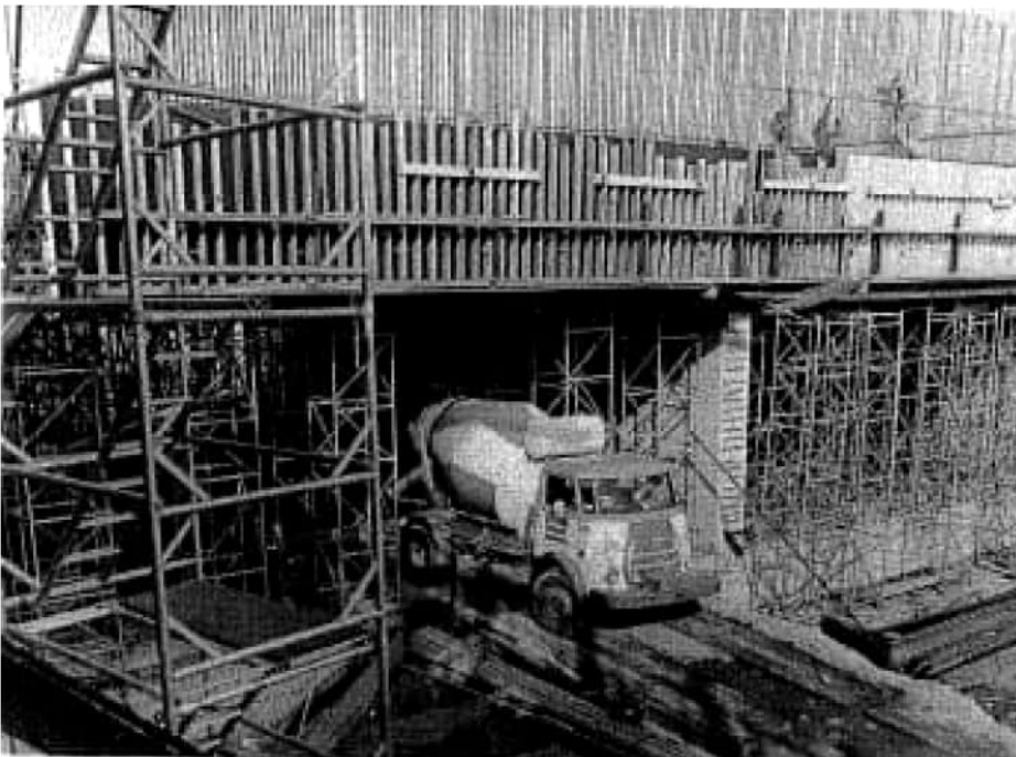
Bekisting dak zinkelement Formwork roof tunnel element
