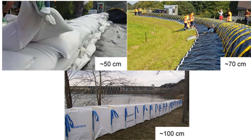
Figure 4-12 Overview of the types of emergency measures included in the scenarios, with the assumed height.
