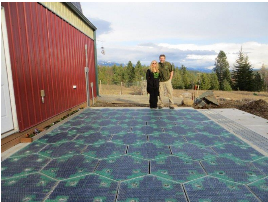
Figure 10: Solar Roadways (Solar Roadways, 2015)
