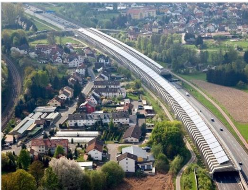
Figure 9: Solar array on roof of noise-barrier tunnel near Aschaffenburg, Germany (U.S. DOT, 2012)
