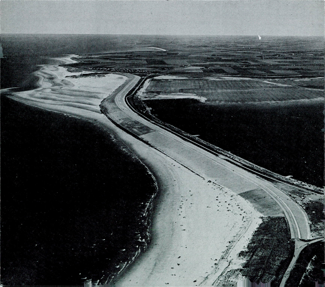
The completed dam in the Veerse Gat
