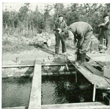
g LEVELLING OF WATERSURFACE AND BOTTOM
