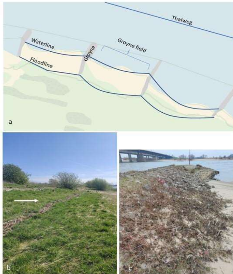
Figure 8. (a) Characteristics of the groyne fields; (b) Picture of a floodline; (c) Picture of a groyne.
